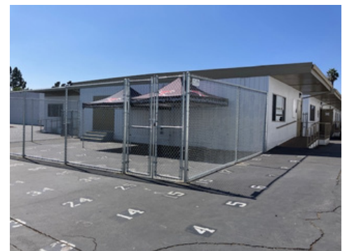
Outdoor yard for dirty work and extra fabrication space
