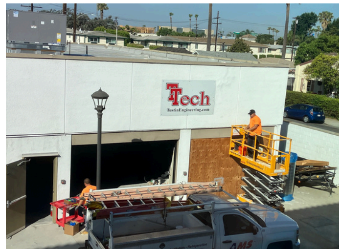
Contractors Finishing Air Conditioning Installation
