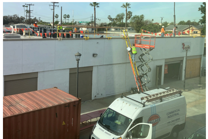
Contractors Working On Roof Repairs
